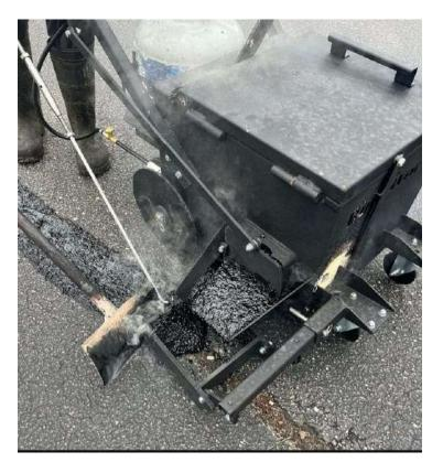
Unlike traditional hot-pour crack sealants, mastic has fine aggregate and polymer added into the material making it load-bearing. It has a reasonable life cycle cost when used to repair and improve ride quality of cupped and wide cracks. This is also a good repair material for deteriorated longitudinal cracks. It requires a high level of care during installation to ensure good ride quality improvement.
