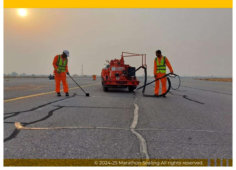
Crack Sealing and filling asphalt concrete pavement cracks is a common road maintenance activity. Specialized materials are placed into or above cracks to prevent the intrusion of water and incompressible material into the cracks and to reinforce the adjacent pavement, Crack Sealing & Filling delays the total reconstruction for several years and thereby saving cost.
