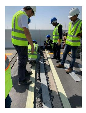
Bridging plates are then immediately placed by centering over the expansion gap and butt jointing to cover the entire joint length and are embedded into the hot Matrix Binder. Use centering pins placed through the holes in the bridging plates and down into the expansion gap to assure proper centering. Bridging plates shall be cut to the appropriate length to cover the entire joint length without overlap.
