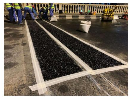
Spread the Binder across joint using a handheld scrapper, immediately remove the masking tape and then immediately apply the Gray Surfacing aggregate.
