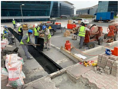
After leveling, additional hot Matrix Binder from the indirectly heated oil jacketed melter is applied to the mixture surface to fill voids.
