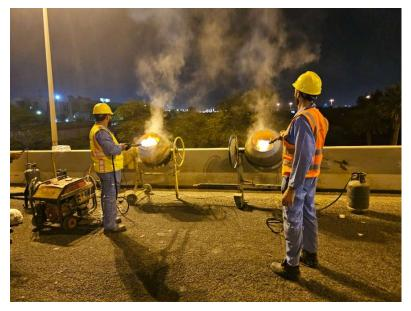
Heated binder is added to the heated Structural Aggregate in the drum mixer or Patcher unit at a ratio of 15 to 20 % Binder. Minor variation in the amount of Matrix Binder added to the heated aggregate is allowed.
