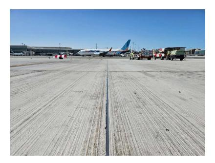
Note: With self-leveling silicone sealants, air voids (bubbles) may develop if pavement moisture content and ambient temperature are high (fresh concrete during hot, humid conditions). Warm ambient temperature increases moisture vapor release. These vapors can migrate through partially cured sealant creating air voids. When sealant has fully cured, no additional voids will develop.
