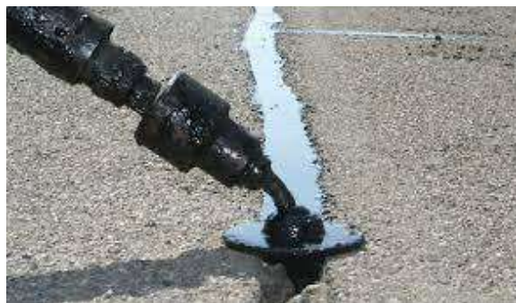
Type: Normal Random Crack Sealing
